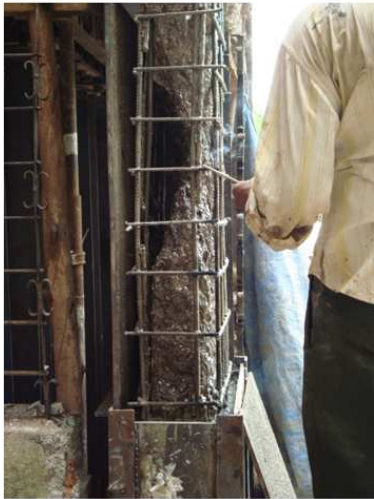
Photograph 6: Steel Plate Jacket
