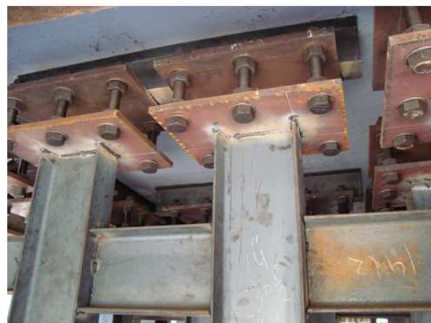
Photograph (5): Props as part of load release system
