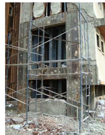
Photograph 8: Completed Steel Jacket Frame
