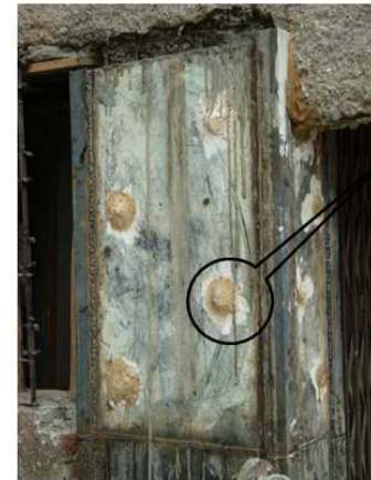
Photograph 7: Provision for high pressure grout
